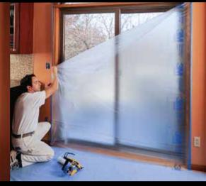
STEP 3: Unfold the film and adhere to the pre-taped side of the door. Tape the top and bottom. NOTE: Cut a small slit for ventilation.
