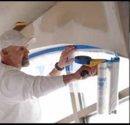
**STEP 2:** Use the 3M<sup>™</sup> Hand-Masker<sup>™</sup> M3000 Dispenser to apply film to the top of the window.
