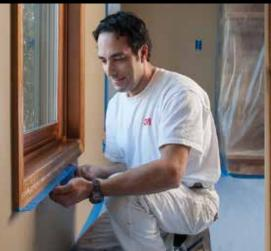
**STEP 1:** Pre-tape the bottom of the window.
