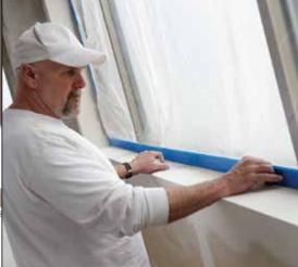
**STEP 3:** Unfold the film down the window and adhere to the pre-taped sides and bottom of the window.
