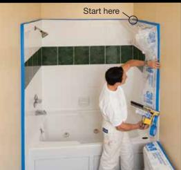
STEP 2: Use the 3M<sup>™</sup> Hand-Masker<sup>™</sup> M3000 Dispenser to apply film to the opposite side of the insert.
