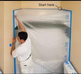
**STEP 3:** Unfold the film and adhere to the pre-taped side of the insert.
