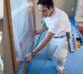
**STEP 3:** Unfold the film and adhere to the pre-taped bottom of the window. Tape the sides.
