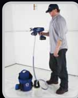
3. Turn on air compressor. Prime sprayer.
