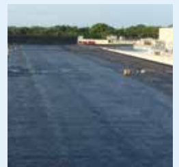
ASPHALT/BUR/ GRANULAR CAP SHEET
