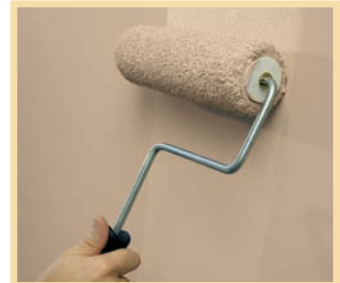
Touch up with the same type of roller cover used to backroll the topcoat.
