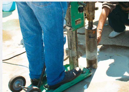
Drilling a core sample
